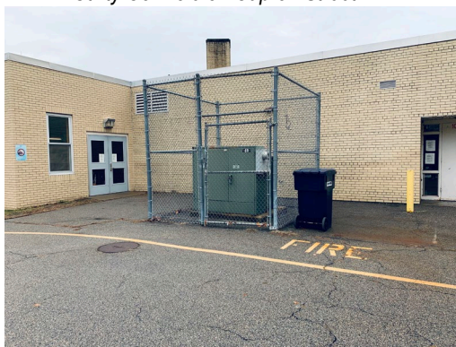
Utility Co. Pad-mount Transformer
