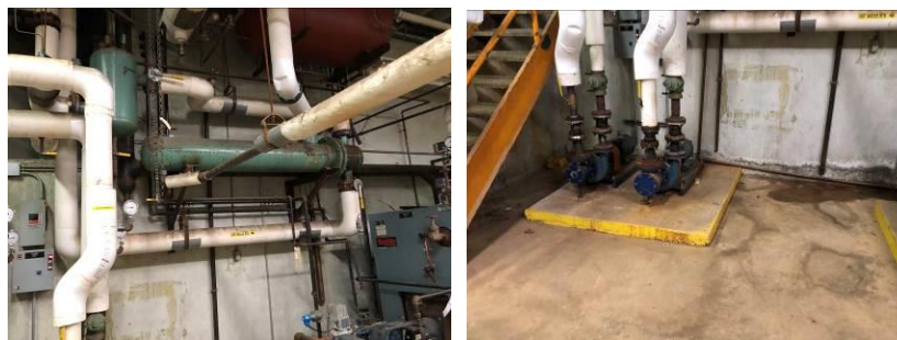
(L - Steam-to-Hot Water Heat Exchanger, R - Hot Water Pumps)
