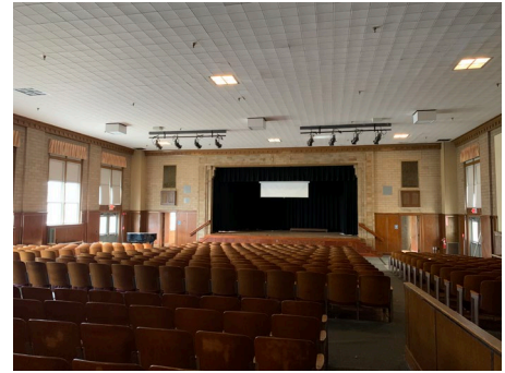
Auditorium surface 1'x4' – 4 lamp fluorescent lensed light fixtures
