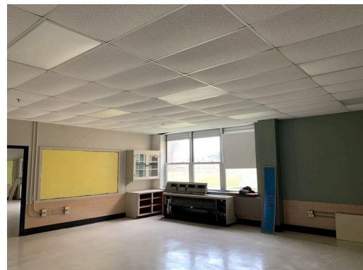
Classroom recessed 2'x4' – 4 lamp fluorescent lensed light fixtures
