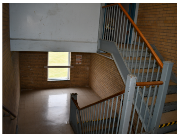
Stairwell at 1936 High School with non-compliant handrails and tread nosings
