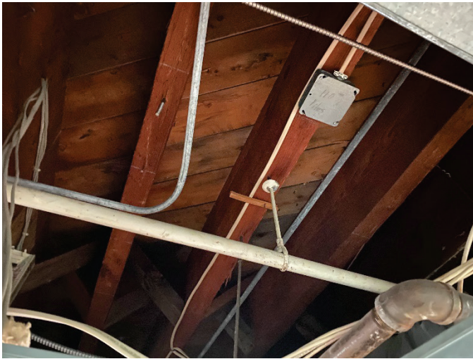
Example Original Building Floor Framing
