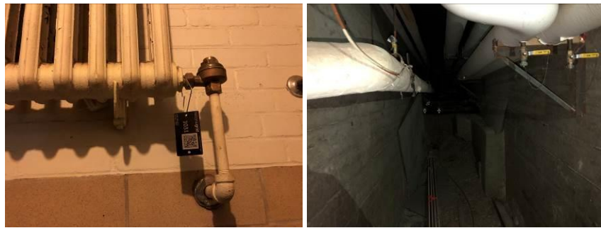
(L - Steam Radiator and Steam Trap, R - Steam Pipe Tunnel)
