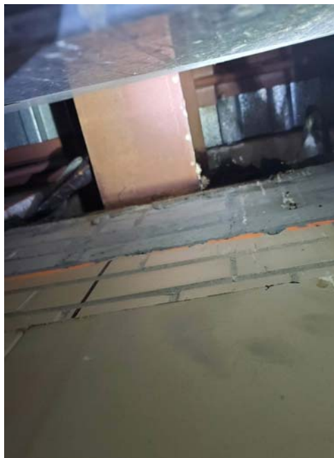
Photograph #2 – Beam From 1988 Addition Bearing on Original Masonry Bearing Wall – 1988 Addition and 1936 Original Structure
