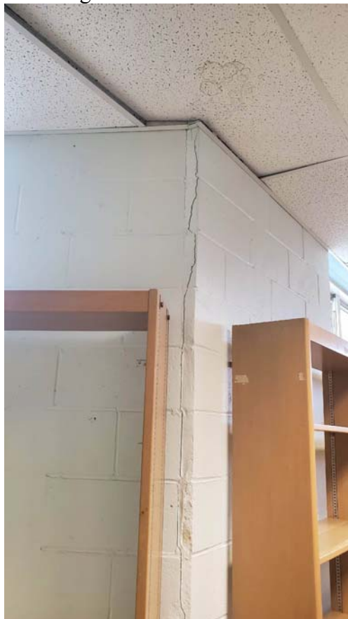
Photograph #8 – Vertical Cracks in Library Masonry Wall – 1988 Addition
