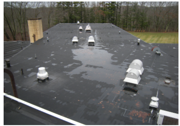
Roof at Junior High School addition with areas of ponding
