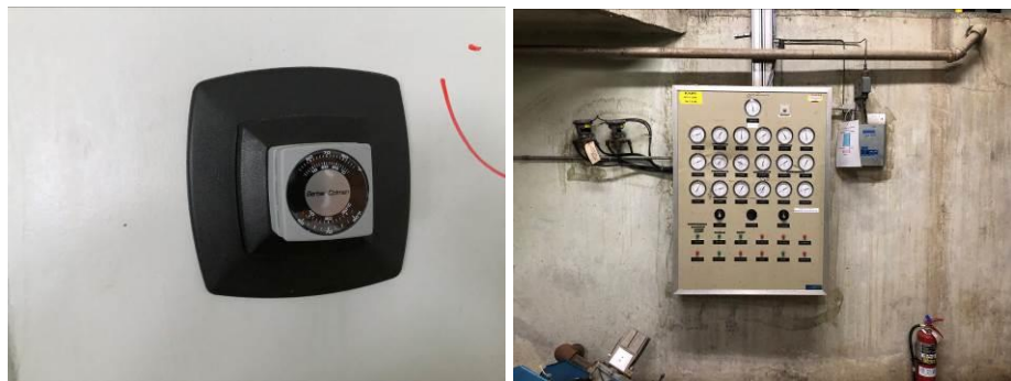
(L - Pneumatic Thermostat, R - Pneumatic Control Panel)
