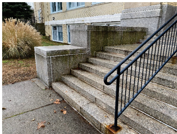
Main Entrance Lacking Handrails on Both Sides of Stair
