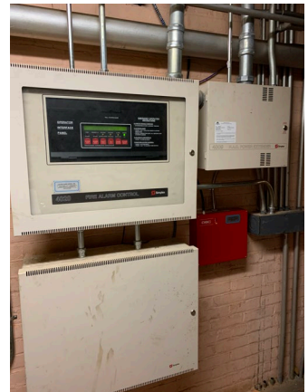
Fire Alarm Control Panel
