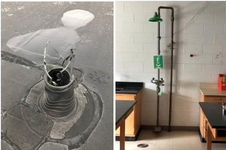
(L - Roof Leak at Damaged Glass Acid VTR, R - Emergency Eyewash/Shower Station)
