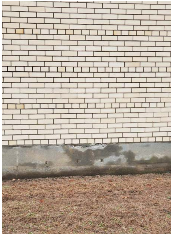
Photograph #15 – Cracked Concrete Foundation Wall – Multiple Locations
