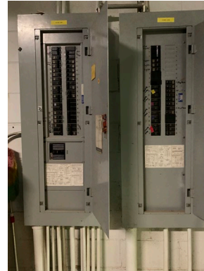
Feeder Circuit Breakers Panels
