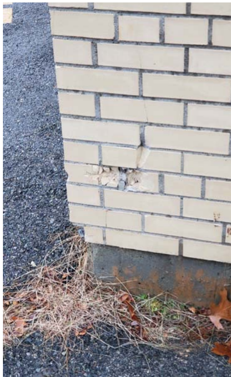
Photograph #12 – Broken Out Masonry in Exterior Wall – Multiple Locations
