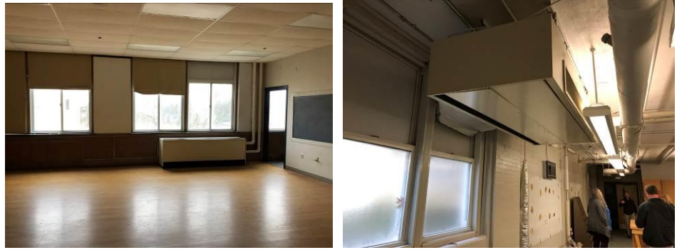
(L - Classroom Vertical Unit Ventilator, R - Classroom Horizontal Unit Ventilator)
