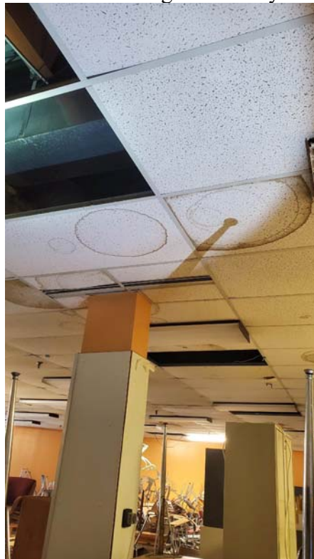
Photograph #10 – Water Damage in “Cafeteria” (1) – 1988 Addition
