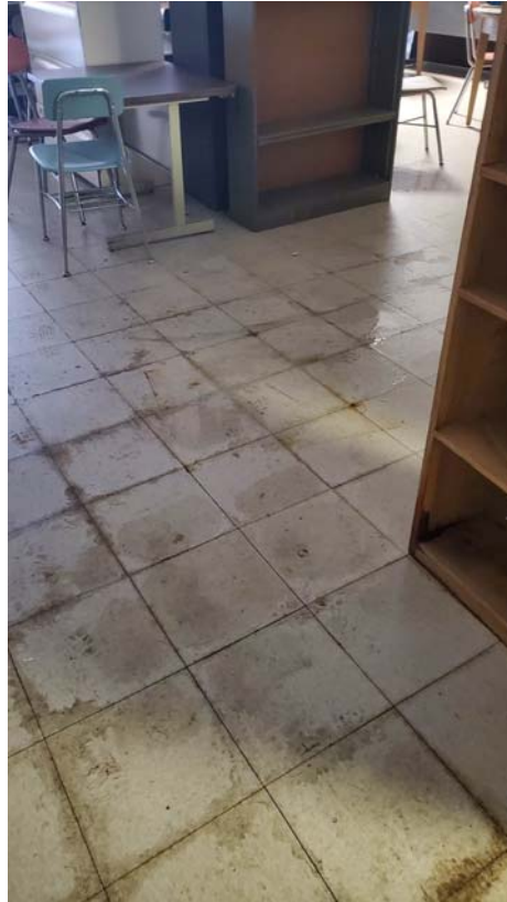
Photograph #11 – Water Damage in “Cafeteria” (2) – 1988 Addition
