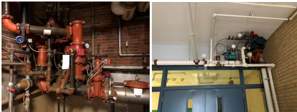
(L - Sprinkler Riser Station, R - Dry Sprinkler Valve)
