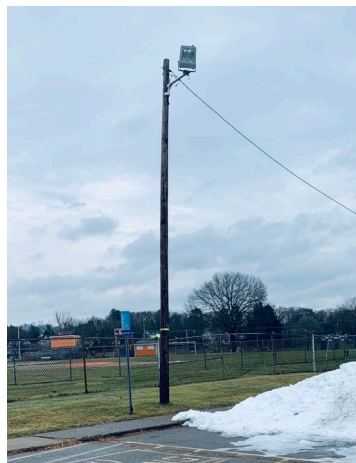
Exterior Flood Light on Utility Co. Pole
