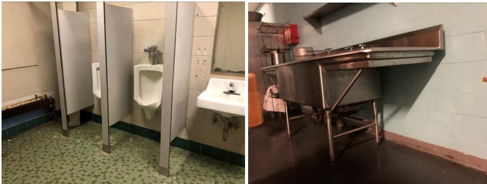
(L - Wall-hung Urinals, R - 2-compartment pot sink without interior grease trap)
