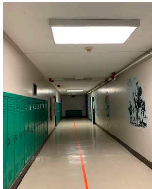
Corridor surface 4'x4' – 4 lamp fluorescent light fixtures
