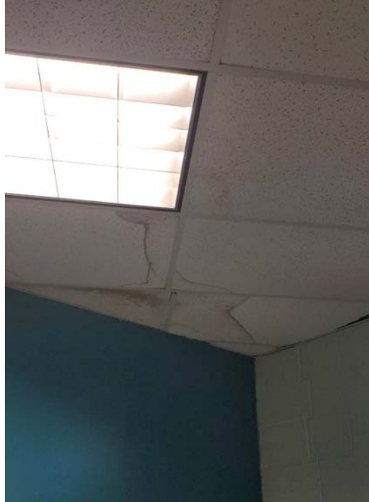
Photograph #9 – Water Damage in Library – 1988 Addition
