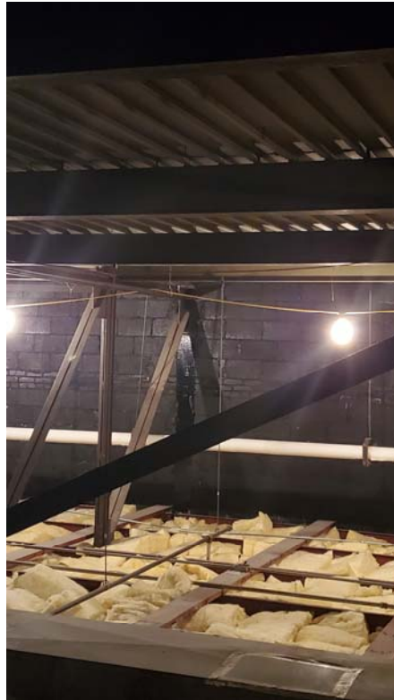
Photograph #1 – Lack of Masonry Wall Ties – 1952 Addition
