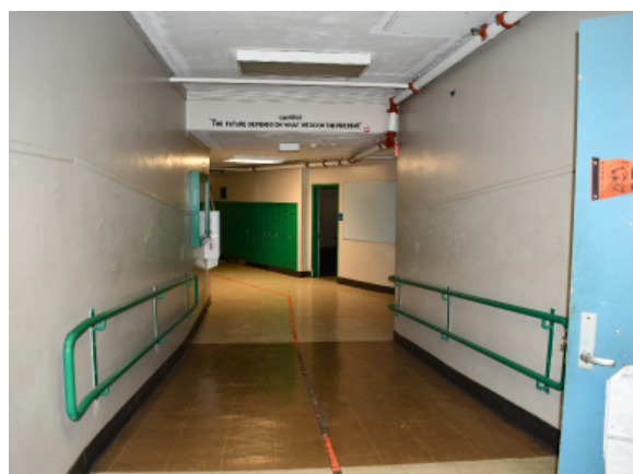
Ramp between 1936 High School and 1952 War Memorial Gym addition with non-compliant slope
