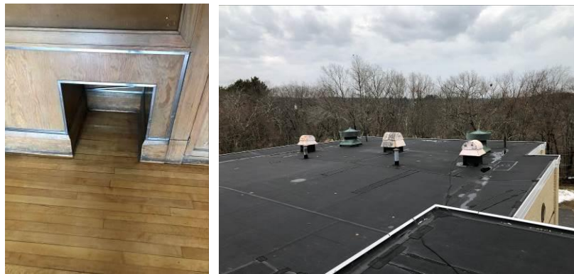
(L - Typical Classroom Exhaust Opening, R - Roof Exhaust Fans)
