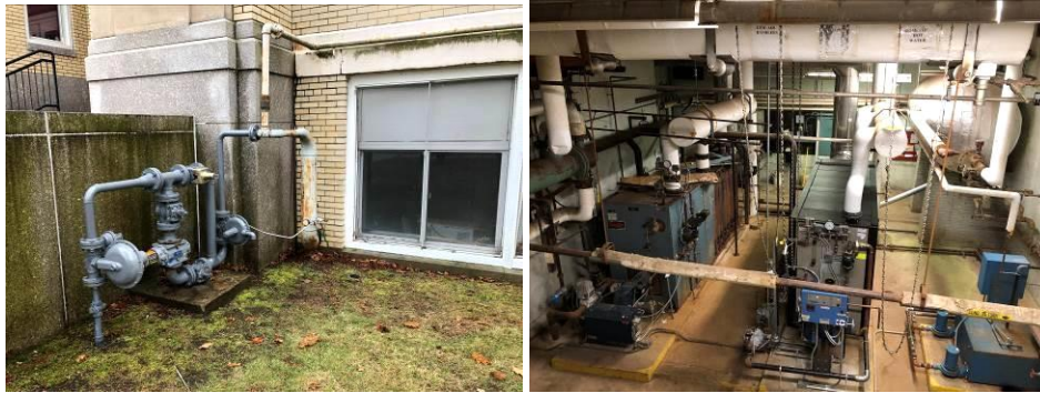
(L - Gas Service and Gas Meter, R - Horizontal Domestic HW Storage Tank)
