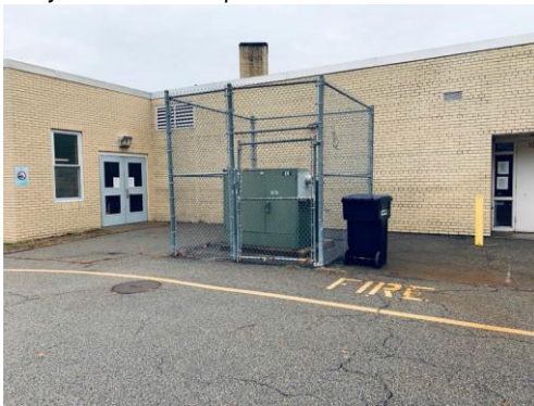
Utility Co. Pad-mount Transformer
