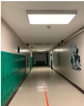
Corridor surface 4'x4' – 4 lamp fluorescent light fixtures
