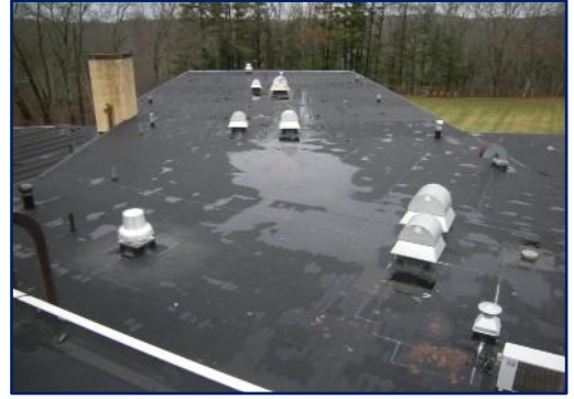
Roof of Junior High School addition with areas of ponding
