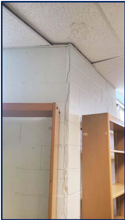
Photograph #8 – Vertical Cracks in Library Masonry Wall – 1988 Addition
