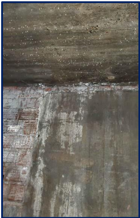
Photograph #4 – Cracked Concrete and Deteriorated Masonry in an “Unexcavated” Room – 1936 Original Structure
