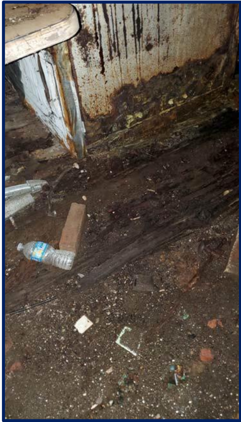
Photograph #3 – Water Damage in an “Unexcavated” Room – 1936 Original Structure
