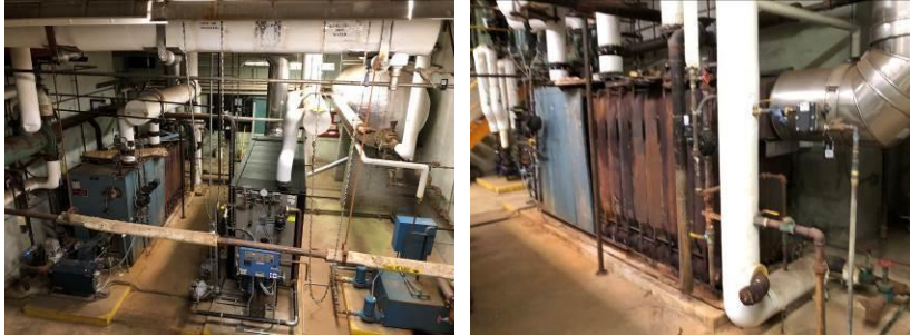
(L - Steam Boilers B-1 and B-2, R - B-1 cover removed)
