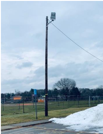
Exterior Flood Light on Utility Co. Pole
