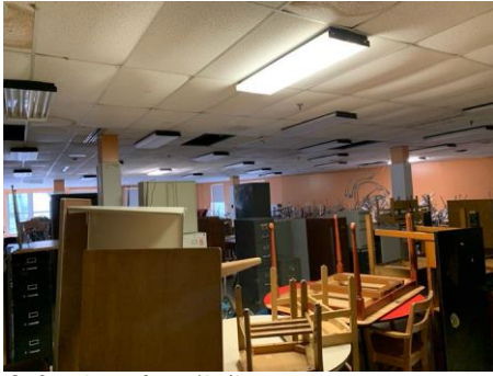
Cafeteria surface 1'x4'- 4 lamp fluorescent lensed light fixtures
