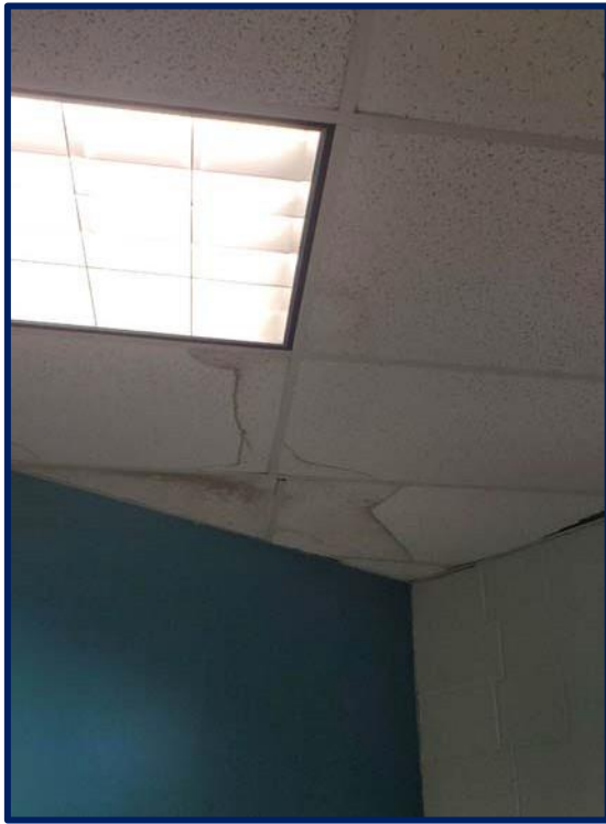
Photograph #9 – Water Damage in Library – 1988 Addition
