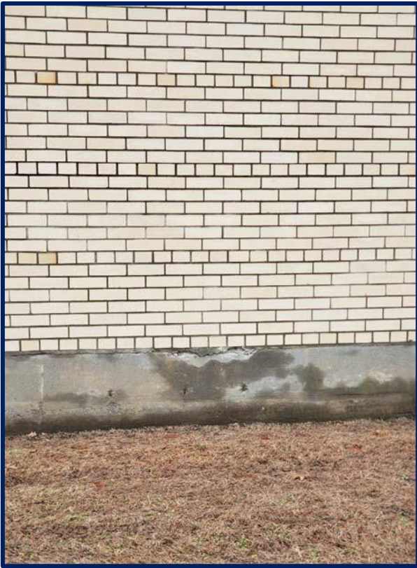
Photograph #15 – Cracked Concrete Foundation Wall – Multiple Locations
