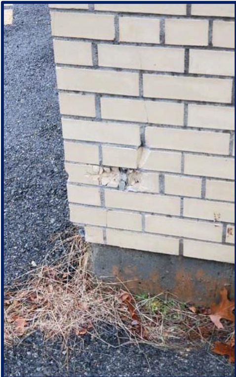
Photograph #11 – Water Damage in “Cafeteria” (2) – 1988 Addition
