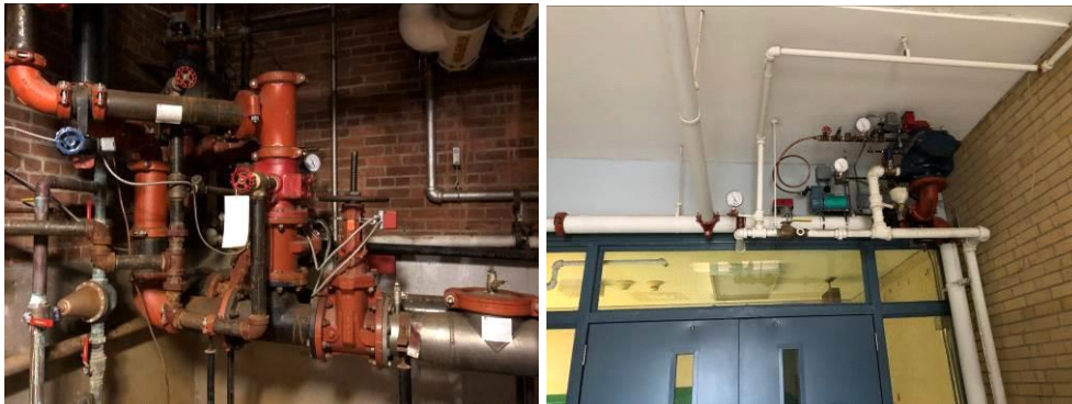
(L - Sprinkler Riser Station, R - Dry Sprinkler Valve)
