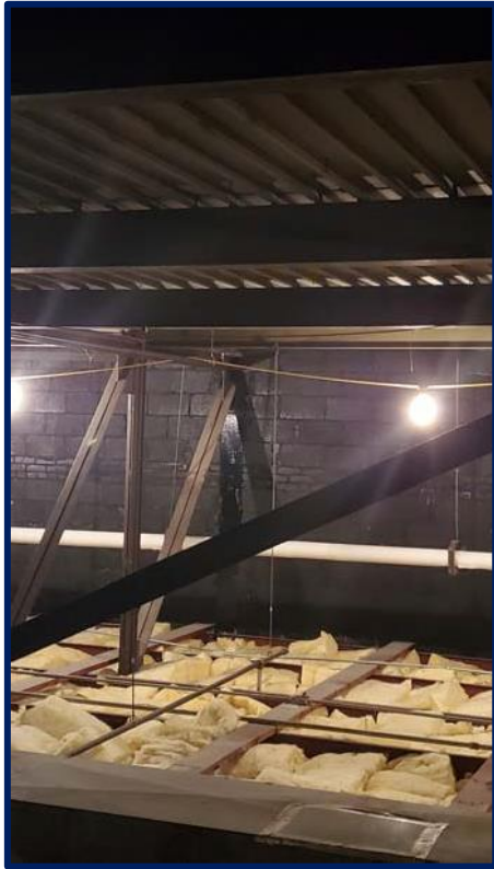
Photograph #1 – Lack of Masonry Wall Ties – 1952 Addition
