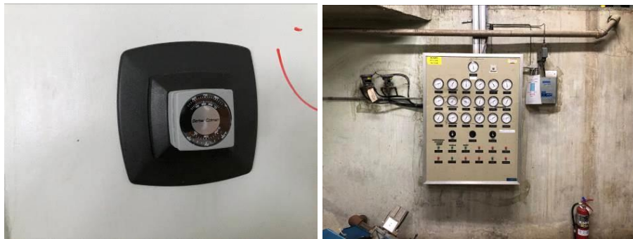
(L - Pneumatic Thermostat, R - Pneumatic Control Panel)
