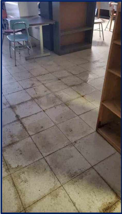
Photograph #11 – Water Damage in “Cafeteria” (2) – 1988 Addition
