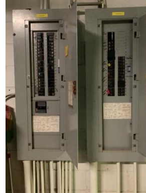
Feeder Circuit Breakers Panels
