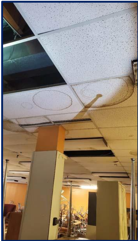
Photograph #10 – Water Damage in “Cafeteria” (1) – 1988 Addition
