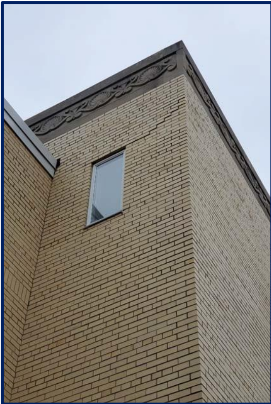
Photograph #14 – Shifting Masonry in Exterior Wall – Multiple Locations
