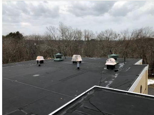
(L - Typical Classroom Exhaust Opening, R - Roof Exhaust Fans)
