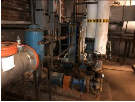
Hot Water Pumps P-1 and P-2
