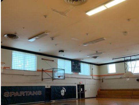
Gymnasium surface 1'x4' – 6 lamp T5 fluorescent light fixtures with cages
