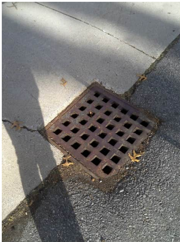
CB-1669: CB located in house #24 sidewalk/driveway – bypass likely
