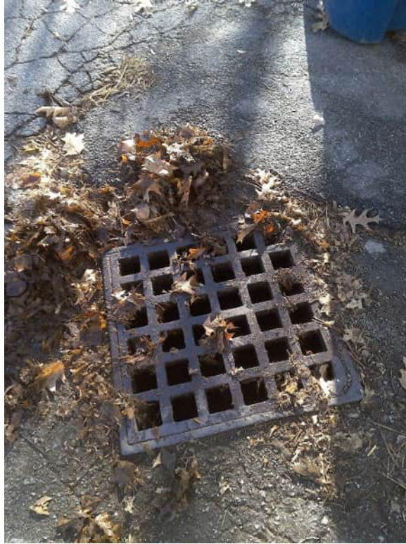
CB-1668: CB located in middle of house #31 driveway entrance – bypass likely
