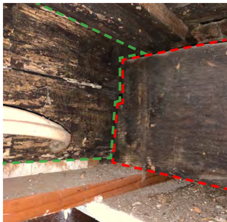
Fig. 66 - Kitchen ceiling removed above bake oven showing joint of west chimney girt (red) to the east/west girt above the fireplace wall (green). Whitewash on the latter suggests it was originally exposed to view
