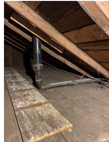
Cast iron vent (Attic)
