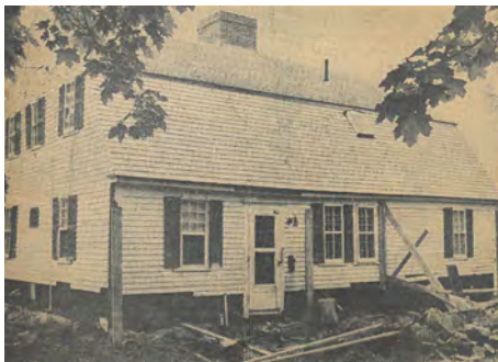
Fig. 8 – 1972 photo from the Worcester Evening Gazette showing the house mid-restoration. Selective sill repairs and re-painting are mentioned in the article. Courtesy of Uxbridge Historical Society
