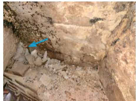
Fig. 34 – Original kitchen stone fireplace jamb wall above jamb of current fireplace at lower left. Blue arrow points to gudgeon for crane in stone jamb
