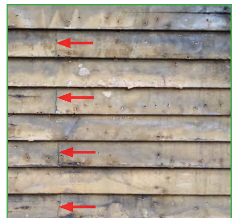
Fig. 20 – Original (ca. 1791) lapped siding at Memorial Hall in Charlestown. Note that horizontal intersections between boards (red arrows) are barely visible by virtue of their 'skiving,' or scarf joints
