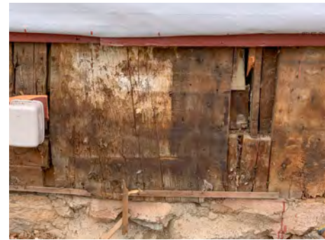
Fig. 40 - Deteriorated plank bottoms exposed during exploratory
