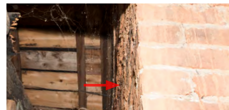
Fig. 27 – Spalling (red) at attic portion of chimney
