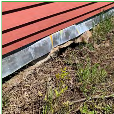
Fig. 30 - Continuous drip cap installed during exterior restoration of 1725 Davis & Abigail Tilden House in Canton.
