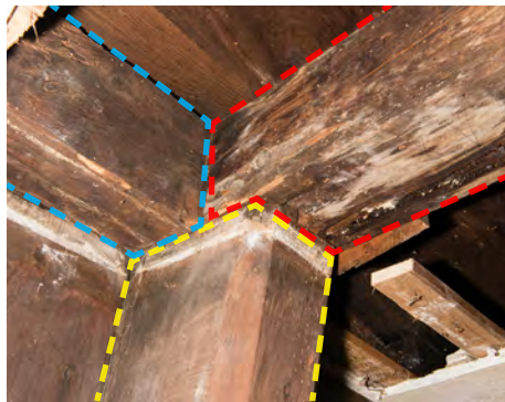
Fig. 65 - Kitchen ceiling removed showing original joint of jowled post (yellow) to north wall plate (blue) and westerly chimney girt (red)
