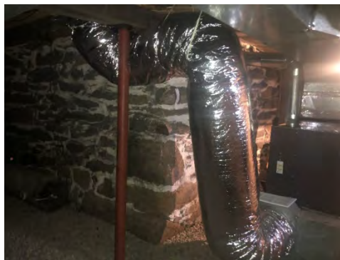
Basement – Furnace Return Air Flex Ductwork
