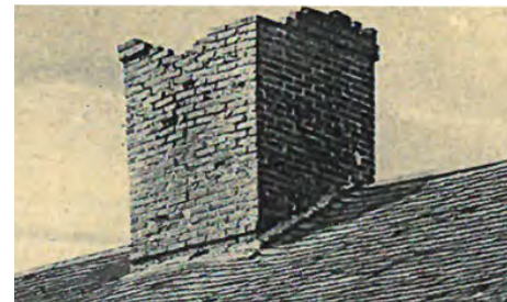
Fig. 25 – Detail of chimney in ca. 1920 photo showing it to be in very poor condition
