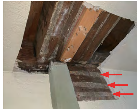
Fig. 47 - Modern plaster removed from ceiling summer beam and wall plank in room 106. Marks from the original plaster (red arrows) on the plank extend to the underside of the beam indicating the room never had a cornice
