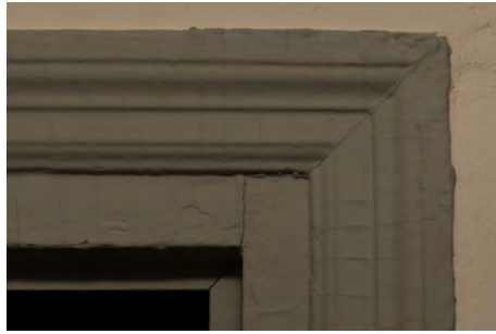
Fig. 50 - Typical original moulded door casing
