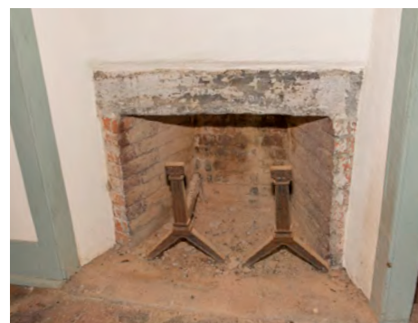
Fig. 36 – The second floor west chamber fireplace that, unlike the brick fireplaces at the first floor, appears to be original to the house
