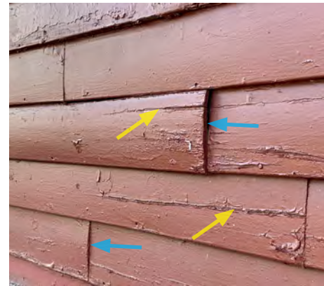
Fig. 18 – A close-up of clapboard siding, showing some dramatic 'cupping' (blue arrows) and splitting (yellow arrows) resulting from long-term exposure to the elements
