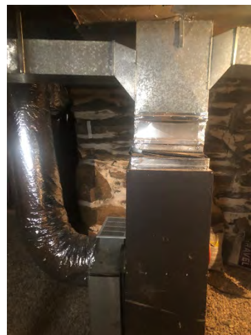
Basement - Existing Oil-Fired Warm Air Furnace
