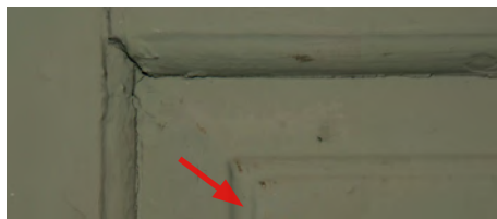
Fig. 54 - Door #17 is an older two-panel door with a bead (red arrow) on the panel edge reused ca. 1770
