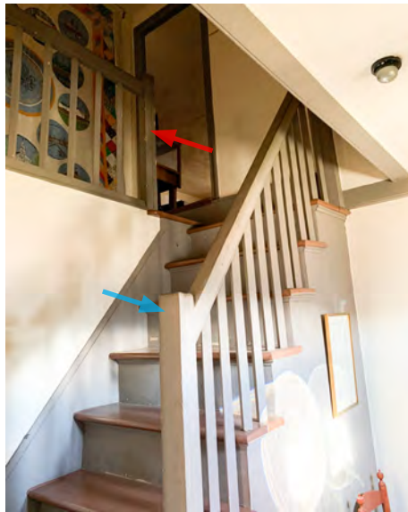
Fig. 59 - The front stair appears to be a well-executed reconstruction of the original, probably dating to 1927. The new railing and newel post (blue arrow) were modeled on the original assembly at the landing (red arrow)
