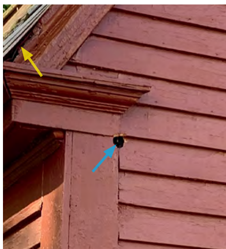
Fig. 23 – Northwest cornice return, showing one of several woodpecker holes (blue); and the rake, which is missing a piece near its intersection with the return (yellow)
