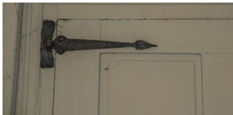
Fig. 53 - Typical mid 19 th -century 4 panel door having very slightly raised square-edged panels set in square-edged rails and stiles. The strap hinge is a 1920s reproduction
