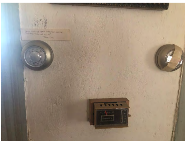
First Floor Thermostats – Furnace Control (left), Entryway Heater Control (Center), Perimeter Electric Radiation Heating (Right)
