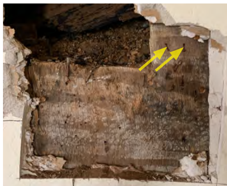
Fig. 46 - Plank wall above the fireplace in room 106 with modern plaster removed showing white stains from original plaster on riven lath. Arrows mark wrought nails from riven lath
