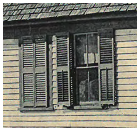
Fig. 12 – Window frames installed in ca. 1900 with 2/2 sash and louvered shutters. The casings are flush with the clapboards.
