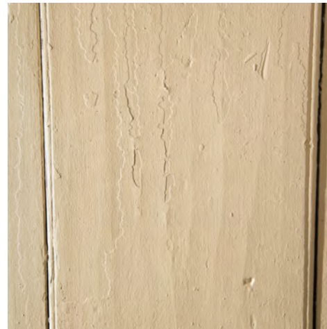
Fig. 62 – Detail of Door #12 showing the character of typical 18th century planed woodwork
