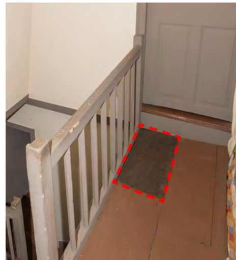
Fig. 69 – Like the rear stair, the front stair and its original landing are painted. A short replacement board (outlined in red) was presumably taken from the attic floor
