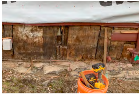
Plank frame exposed by exploratory removal of clapboards
