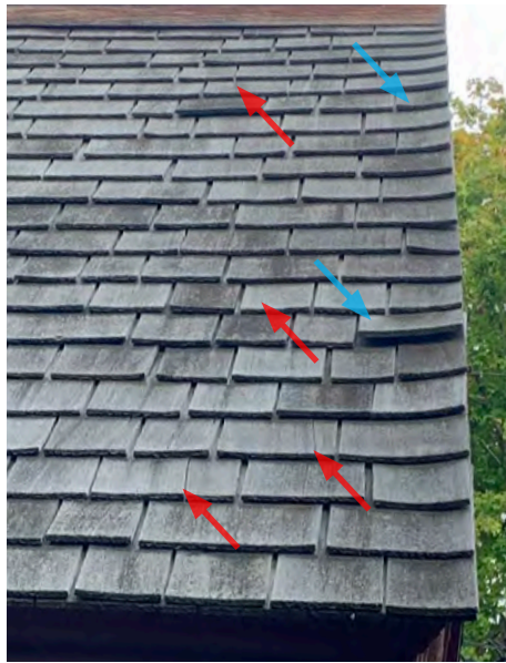
Fig. 21 – Wood roofing shingles are in fair condition, having been replaced just over a decade ago. Only some are split (red) and cupping (blue) while many show mild warping
