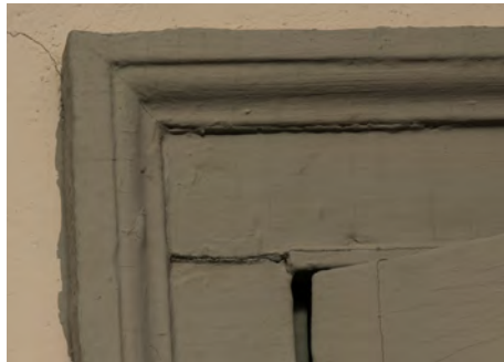
Fig. 51 - Original flat casing with ogee band molding on an original board-and-batten door (Door #5)
