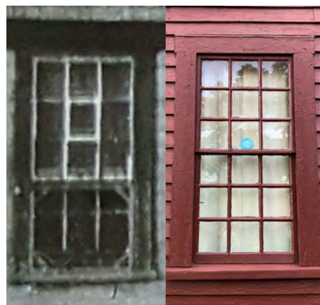
Fig. 10 – Original 9/6 sash layout on the left compared to 9/9 1927 sash on the right
