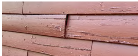
Long, sawn clapboards are more likely to warp with age
