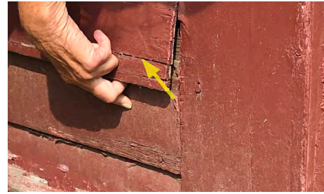
Fig. 17 – A clapboard that has loosened near its intersection with the corner post. Note splitting (yellow arrow)
