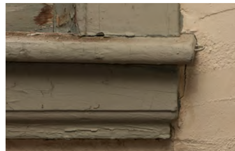
Fig. 56 – Typical window casing that likely dates to installation of 2/2 windows ca. 1900
