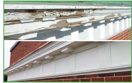
Fig. 24 – Before and after images of epoxy consolidated wood cornice at Newburyport High School
