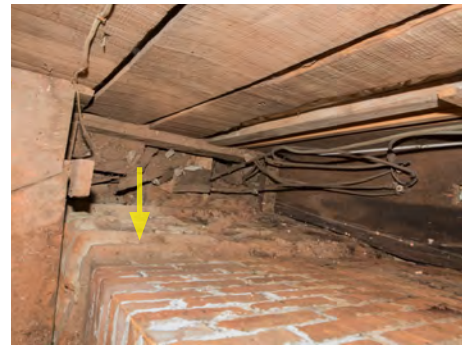
Fig. 33 – Yellow arrow points to transition of chimney from stone to brick about 2' above 2nd floor
