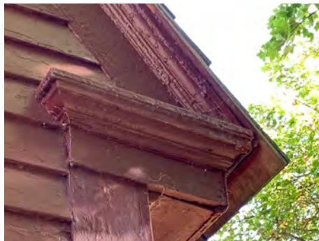
Fig. 22 – Detail of roof cornice, rake boards and cornice return showing molded trim that likely dates to 1927 or earlier
