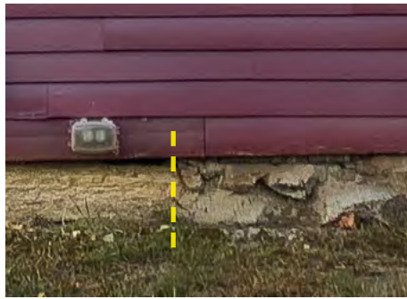
Fig. 29 - Closeup of exterior foundation wall, showing transition dressed granite to fieldstone where the east ell jointed the main house
