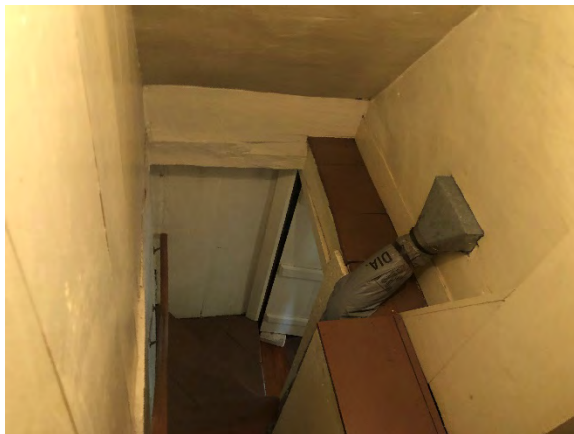
Second Floor Stairwell – Toilet Room Heating Supply Flex Ductwork
