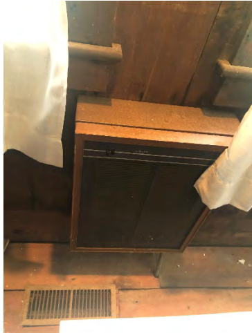
First Floor Entryway - Electric Unit Heaters
