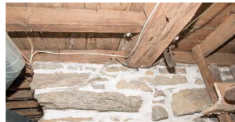
The granite chimney base as seen from the basement
