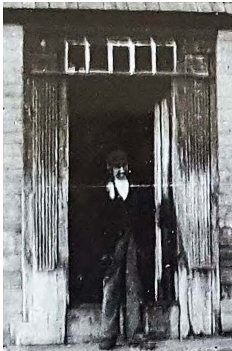
Fig. 14 – Original front entry pilasters and transom lights from late 19 th -century photo
