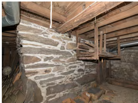
Fig. 31 - An overall photo of the granite chimney base
