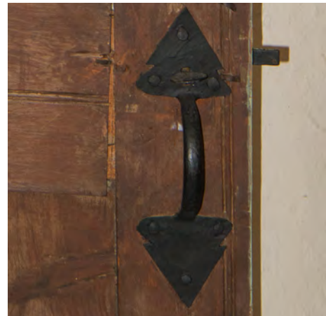
Fig. 55 – Typical reproduction Suffolk latch likely installed in 1927
