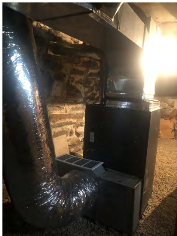
Basement - Existing Oil-Fired Warm Air Furnace
