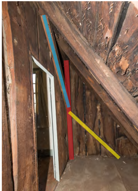
Fig. 44 - The 'over-eave' storage area at the house's south side with the endwall post outlined in red and rising and falling braces in blue and yellow, respectively
