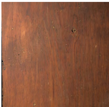
Fig. 61 - Detail of sheathing board on the west wall showing marks from a scraper or plane that are not characteristic of period work
