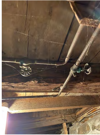
Typical antiquated shutoff valves
