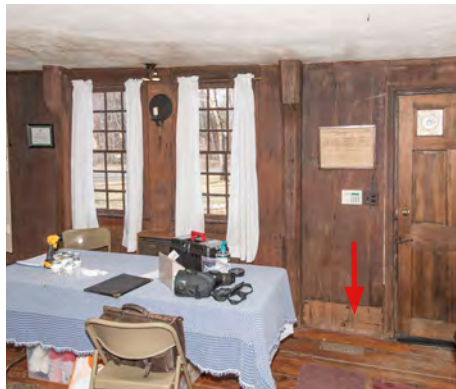
Fig. 60 - The north wall of the kitchen. At other walls, vertical board sheathing extends from floor to ceiling, but here the lower 1' or so has been replaced with a horizontal board (red arrow), likely the result of past sill repairs
