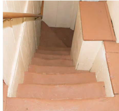
Fig. 68 – The rear stair treads show a weathering pattern typical of well-used stairs wherein the central portions are more worn than the sides due to foot traffic
