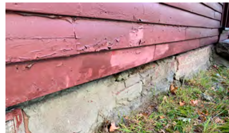
Fig. 19 – A close-up showing dramatic weathering of paint, particularly at lower clapboard courses
