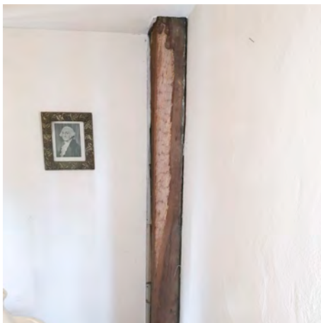
Fig. 39 - First-floor (northwest) corner post with modern casing removed. These corner posts never had braces
