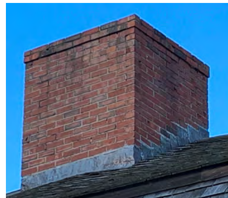
Fig. 28 – Current photo of chimney as rebuilt in the 1970s with new waterstruck brick
