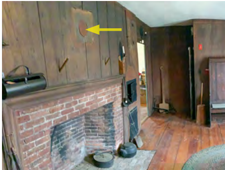
Fig. 37 - The walls over first-floor fireplaces have been punctured to vent freestanding stoves, a practice typical in 19 th and early 20 th -century renovations of earlier homes
