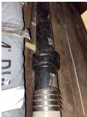
Cast iron - PVC interface
