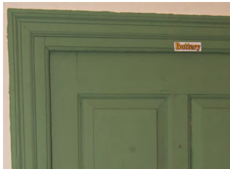
Fig. 52 - Typical original four-panel door with raised and fielded panels
