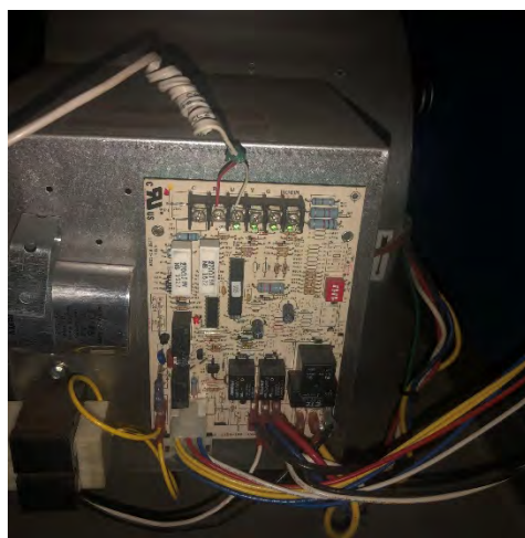
Furnace Controller
