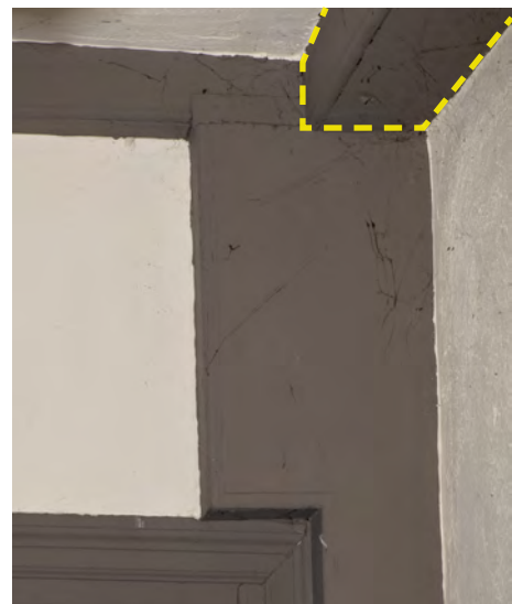
Fig. 49 - Top of jowled post in the entry with original beaded casing fitted over the top of the original door frame. The original beaded casing over the first floor plate is outlined in yellow
