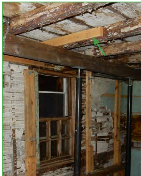
Fig. 67 - The arrow identifies 'sistered' ceiling girt at the 1715 David & Abigail Tilden House in Canton, MA. Leaving the Farnum House's ceilings exposed following structural interventions would expose the repairs and disrupt the building's character
