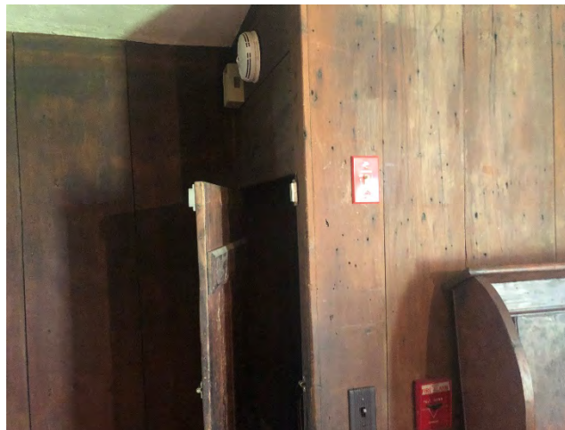
First Floor – Furnace Oil Burner Shut Off Switch
