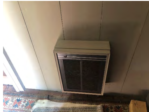
First Floor Entryway - Electric Unit Heaters
