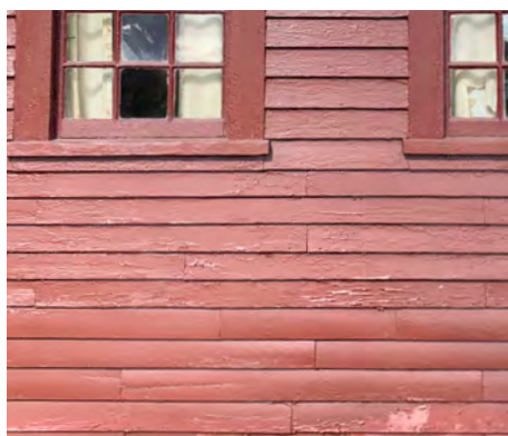
Fig. 16 – Close-up of clapboard siding illustrating typical condition
