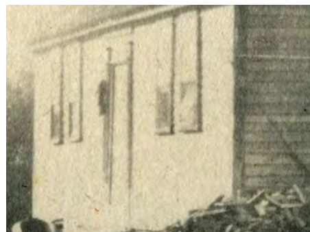
Fig. 11 – Detail from late 19 th -century photo showing the shadow line of the window frames.
