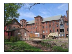
The Stanley Woolen Mill ceased operation in 1988, the last of Uxbridge's textile factories to close. The complex is currently slated for redevelopment, with initial stabilization and upgrades already underway, including oil tank removal, roof repairs, asbestos removal and refenestration. Much of the work is still ahead.
