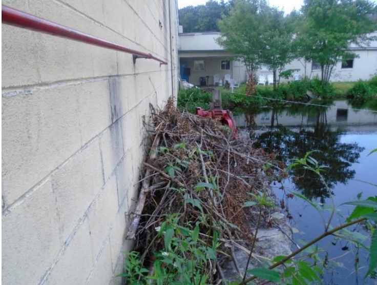
Pile of beaver debris removed from the spillway at Rivulet Village Pond Dam. This was one of multiple piles of debris observed during the assessment.
