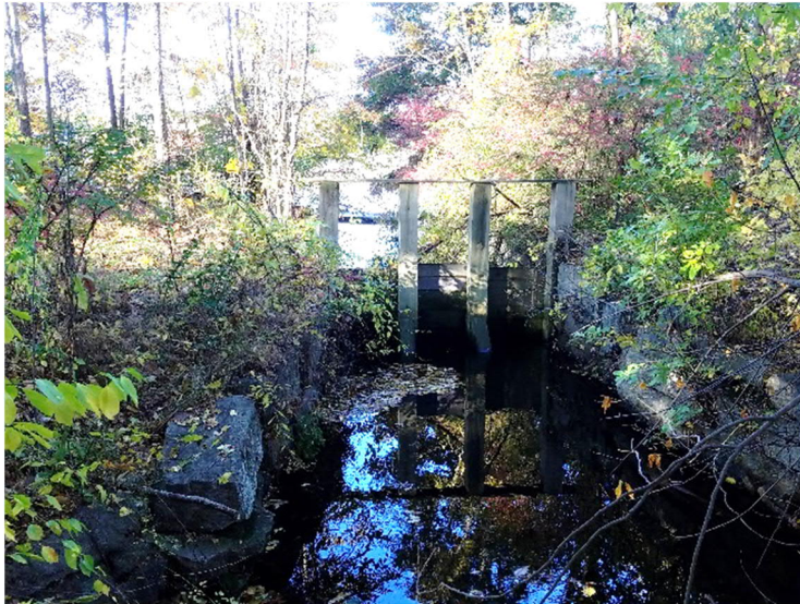
Auxiliary spillway at Whitin Pond Dam.
