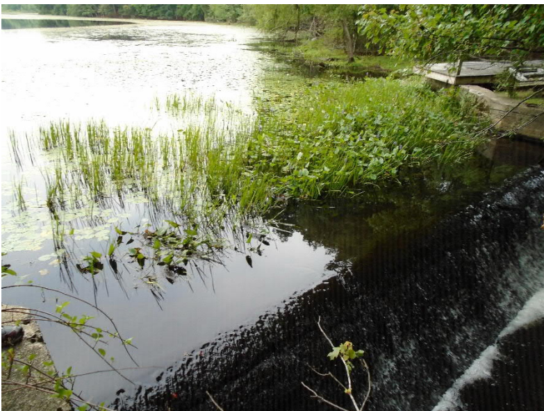
Spillway at Ironstone Reservoir Dam.
