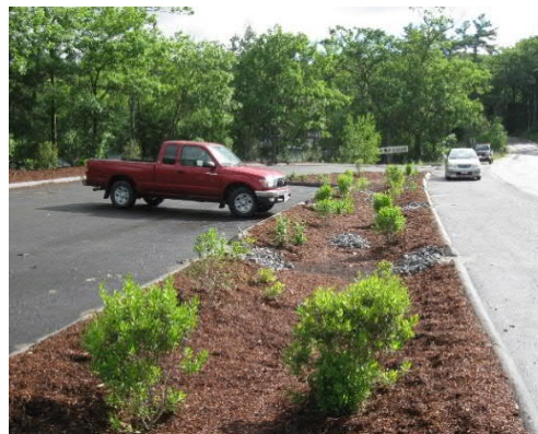
Image 3: Typical parking lot with bioretention and diagram of a bioretention basin. Image source: MA Clean Water Toolkit
