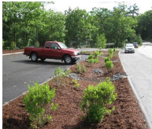
Image 4: Typical parking lot with bioretention and diagram of a bioretention basin. Image source: MA Clean Water Toolkit.
