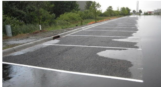
Image 2: Porous asphalt parking lot during a rainfall event. Image source: Potomac Conservancy
