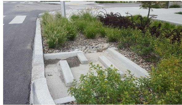
Image 1: Example of an established bioretention basin with a concrete curb cut and concrete pretreatment structure to remove sediment before runoff enters the planted portion of the basin. Image source: Fuss & O'Neill
