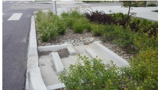
Image 1: Example of an established bioretention basin with a concrete curb cut and concrete pretreatment structure to remove sediment before runoff enters the planted portion of the basin. Image source: Fuss & O'Neill
