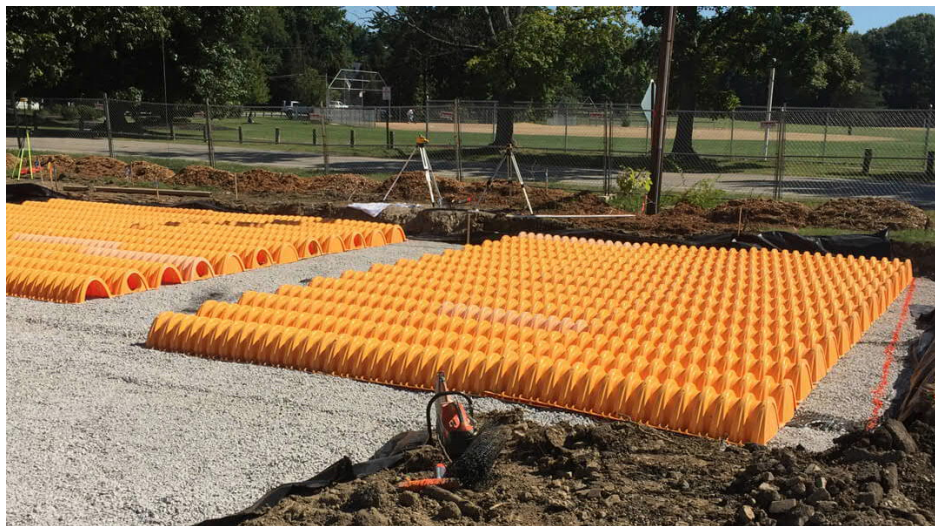
Image 2: Underground infiltration chambers being installed. Image source: StormTech
