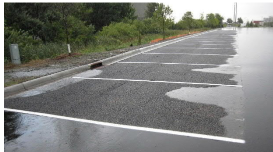
Image 2: Porous asphalt parking lot during a rainfall event. Image source: Potomac Conservancy
