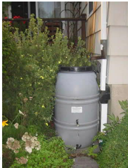
Image 3: Example of an installed rain barrel. Image source: CT DEEP
