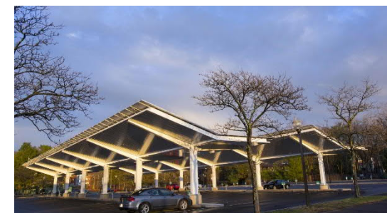
Image 3: Solar Canopy over the parking lot at the Rosham Visitor Center at the University of Massachusetts Amherst. Image source: https://www.umass.edu/sustainability/robsham-visitor-center-solar-canopies
