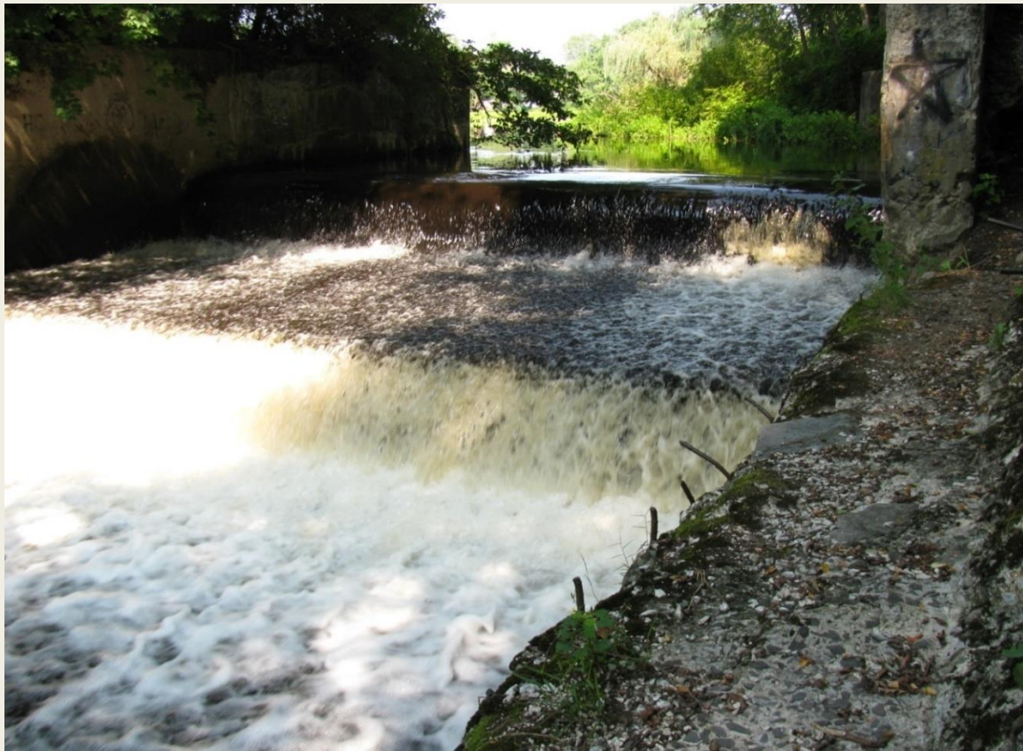
Former State Hospital Dam, Taunton
