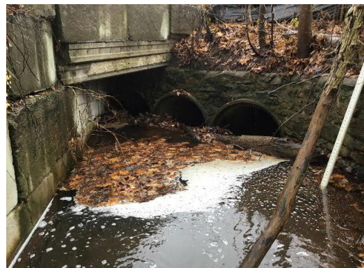
Figure 16. The inlet at crossing xy42069387166088 on Route 16/Douglas Street.
