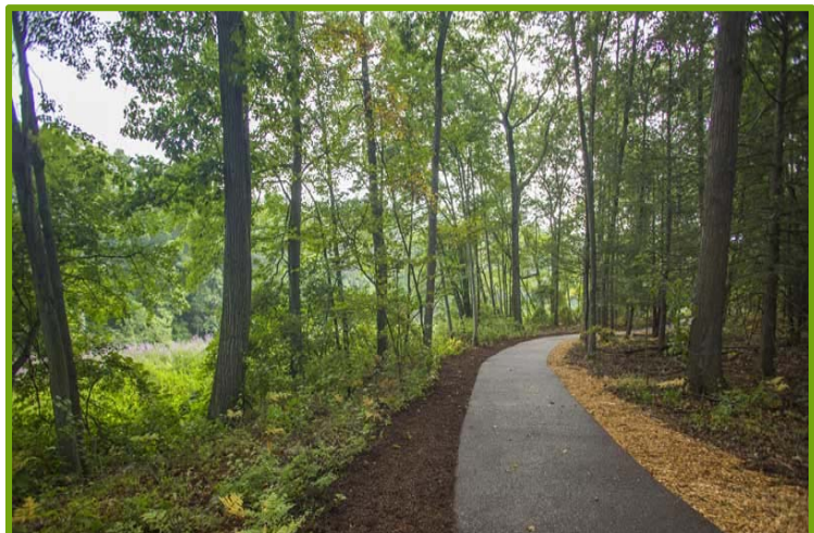
Figure 8 Porous pavement comprised of 50 percent recycled rubber chips and 50 percent chipped granite aggregate at the Wellesley Office Park Walking Path needed to be strong enough to tolerate periodic flooding. (Source: Porous Pave)
