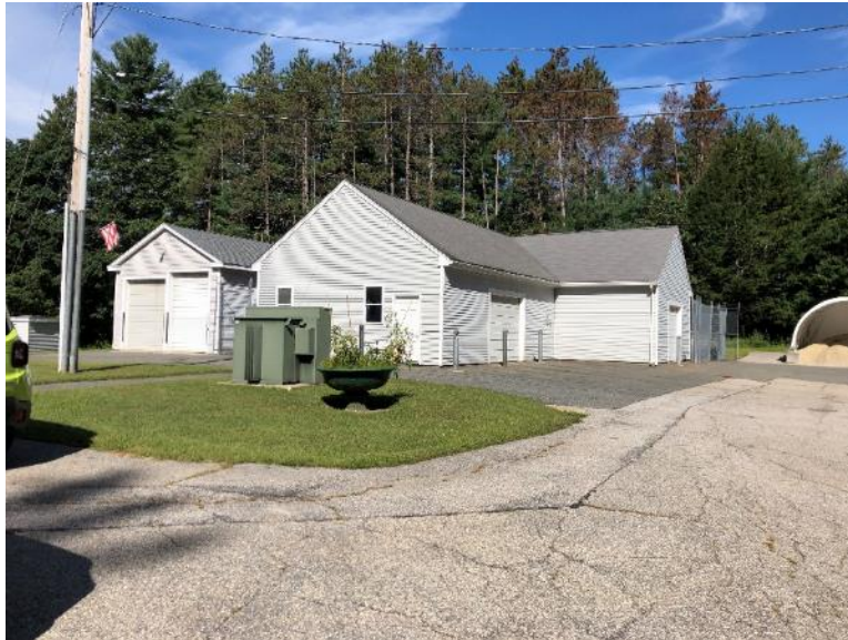
Figure 3-5. Chemical Feed Treatment, Parts Storage and Garage
