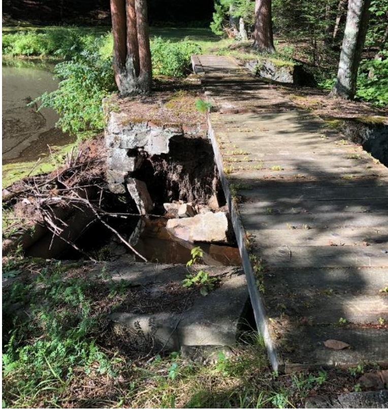
Figure 3-4. Blackstone Well 1 Access Bridge and Dam
