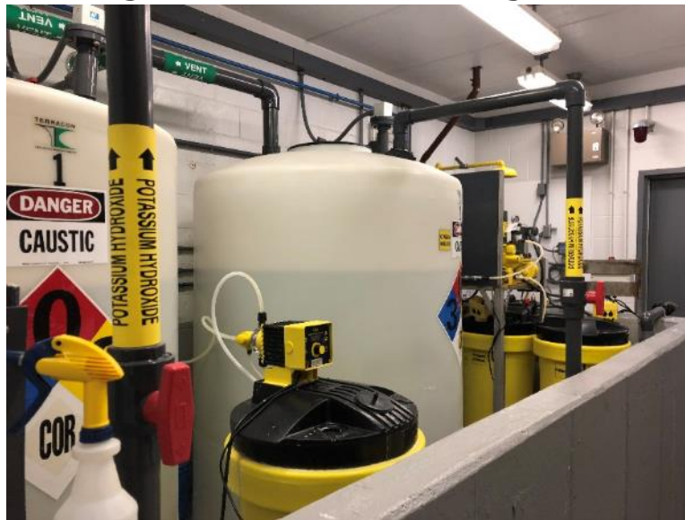
Figure 3-14. Bernat Chemical Storage Area
