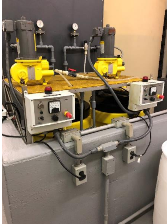
Figure 3-6. Potassium Hydroxide Chemical Feed System
