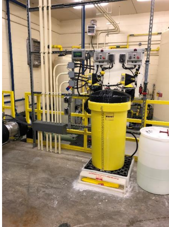
Figure 3-18. Phosphate Feed System
