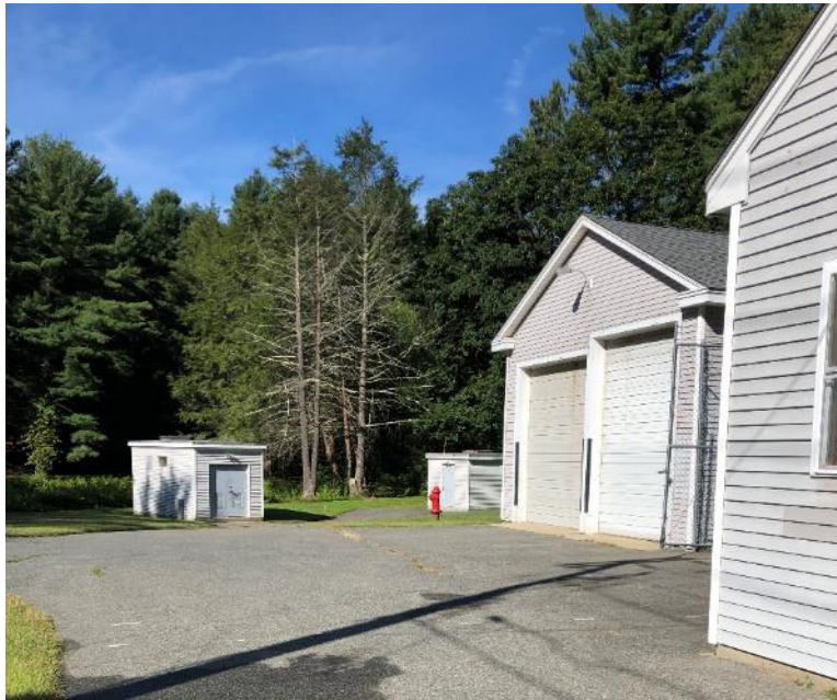
Figure 3-1. Blackstone Wells 2 and 3 and Garage
