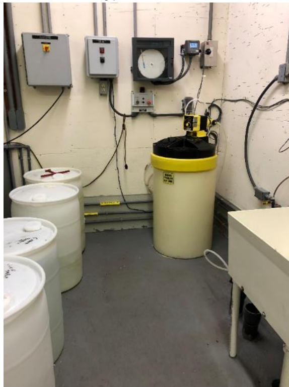
Figure 3-7. Sodium Hypochlorite Chemical Feed System
