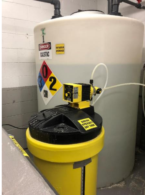
Figure 3-15. Bernat Chemical Storage Area
