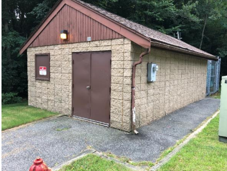
Figure 3-23. Farfard Booster Pump Station Exterior
