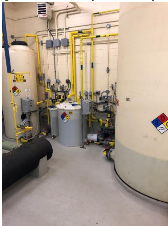
Figure 3-20. Potassium Hydroxide Feed System
