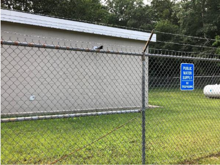
Figure 3-12. Bernat Chemical Treatment Facility
