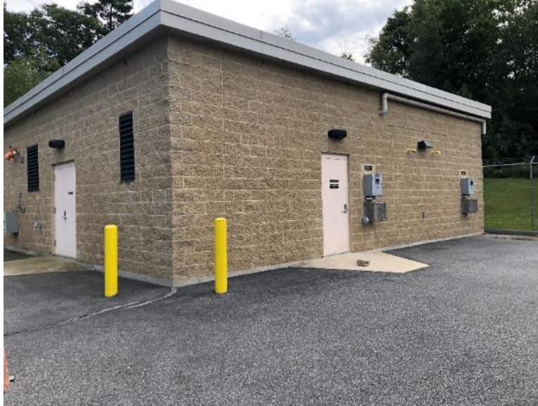
Figure 3-16. Rosenfeld Well Pump Station Exterior
