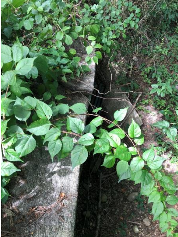
Figure 3-11. Bernat Pump Station Access Drive Culvert
