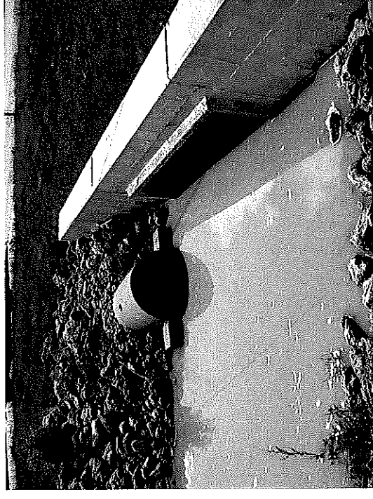
Example of an inundated outfall: the water from the waterbody is backing up into the structure.
